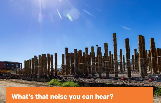
Our build partners are piling the ground in Northcote to prepare for the much-needed foundational wooden poles drilled through the ground to provide structural strength for a building.
