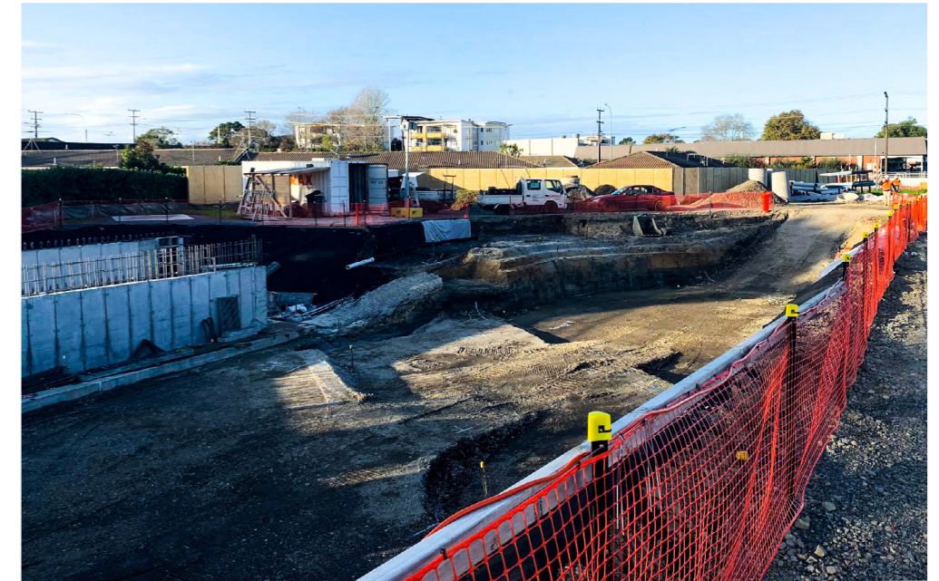
Above Digging and foundation works on the reserve's wetlands area is almost complete
